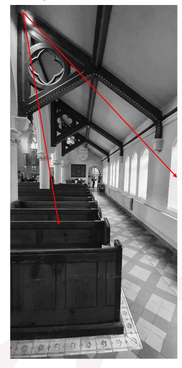
We propose that luminaires are located using the Apex position to the East of each of the beams. From this position a good level of ambient downlighting ahould be achieved, however it is also important to illumaint ethe façade of the Church.
