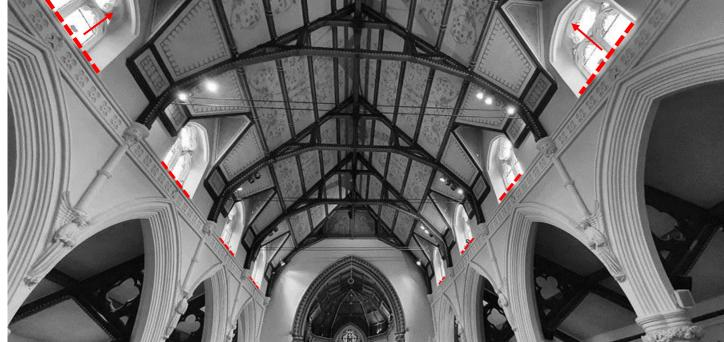
We propose linear LED profile located to each of the lower Clerestory Reveals. These fittings should have a linear distribution to illuminate the window reveal only and not spill into the roof.
