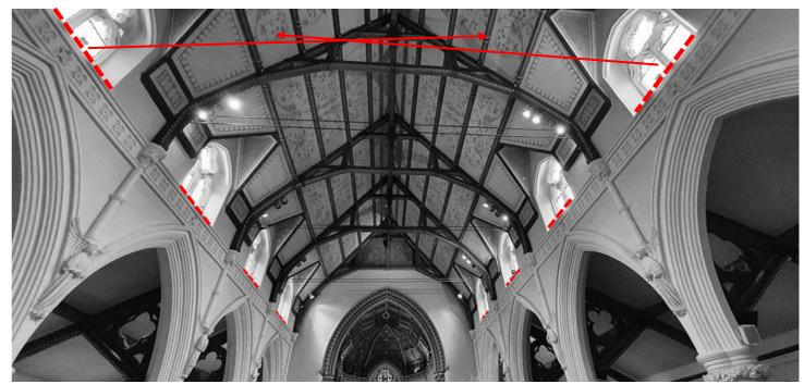
Similarly, to the Clerestory reveals, to capture the Nave roof we propose Linear LED Profile, however these luminaires will be positioned to light the opposing roof section thus avoiding shadowing from the Perlin beams and creating an even consistency to appreciate the detailed painting.
