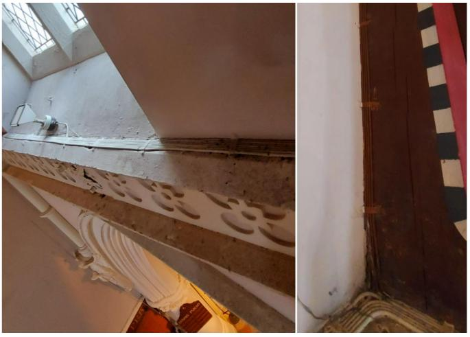
Existing wiring that enters Nave at high level is in good condition and will be utilised. At this point, new wiring will be connected and extended along the Nave cornice to each window and truss beam. The wiring routes will be exactly the same as existing (see image above).
